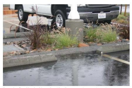
Example of parking lot bioswale with adjacent pervious paving strip
