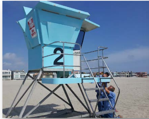
Seasonal installation of Lifeguard Towers and year-round maintenance
