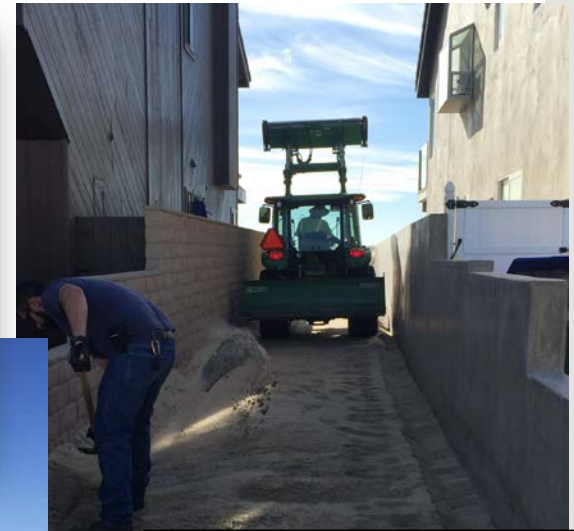
Clearing of easements
