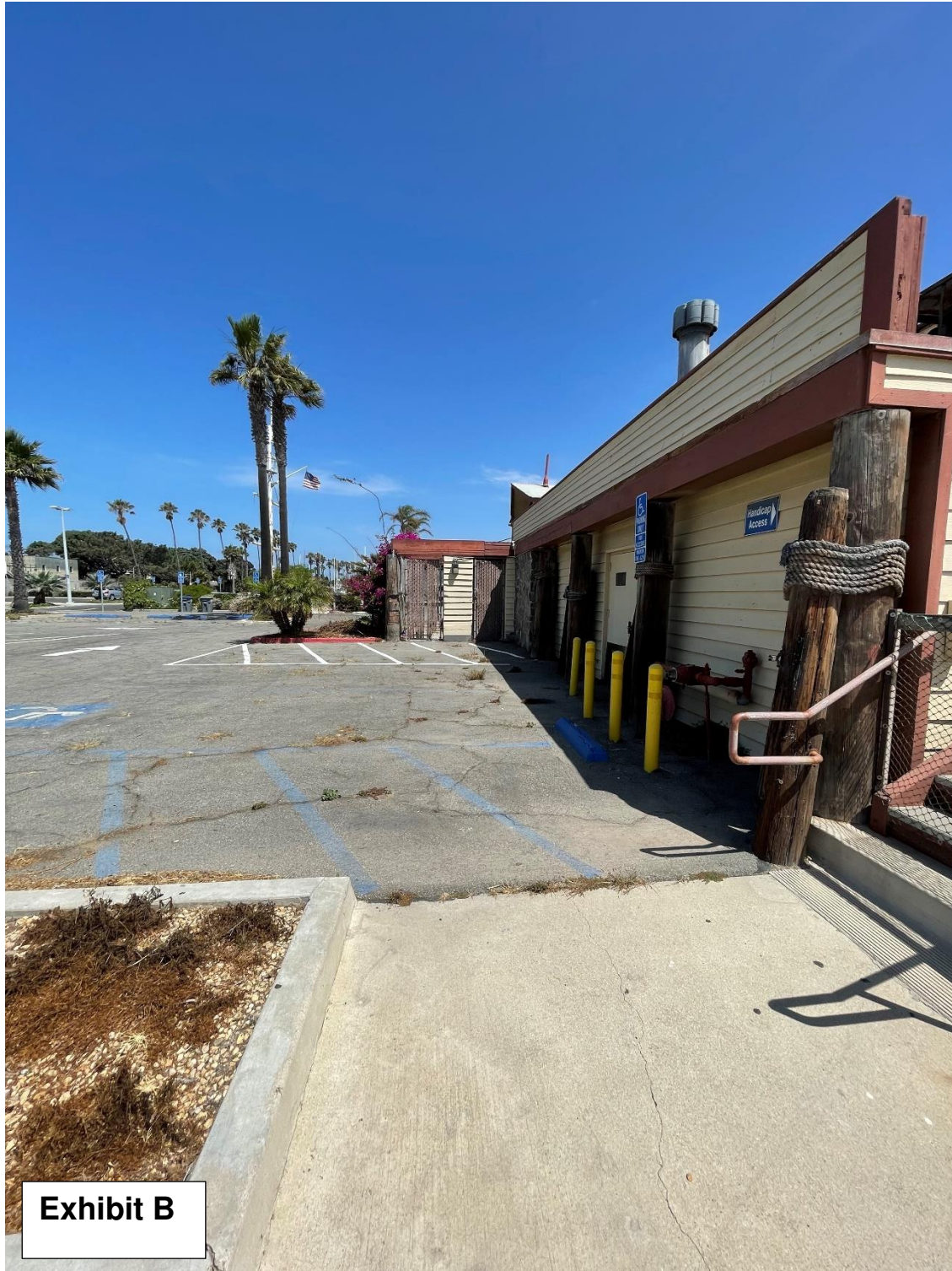
West side of building and parking/loading area looking north.
