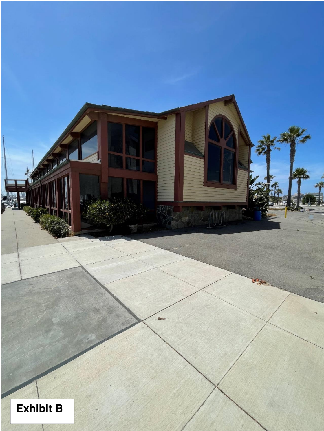
North and east side of building with promenade.
